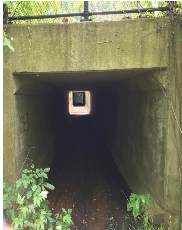
Wildlife crossing underpasses installed along Fairfax County Parkway by Fort Belvoir. This larger box culvert on the parkway is near John J Kingman Road; Right: The smaller box culvert on the parkway is approximately 0.25 miles to the east of the larger one.
