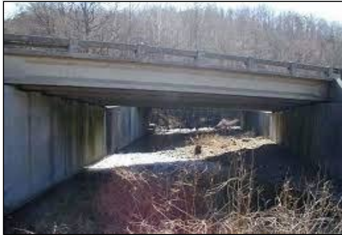
Figure 2-13. Bridge underpass along I-81 north of Buchanan used as a wildlife crossing. (VTRC 2022)
