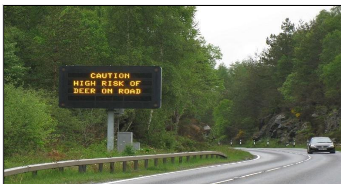
Figure 2-14. Typical changeable message sign to warn drivers of high risk of deer collision. (Johnogroat Journal)
