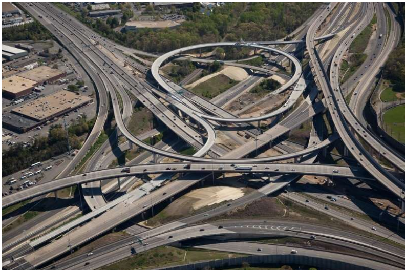
Springfield Interchange Photo Credit: VDOT
